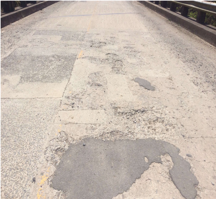
PHOTO 1 Description Deck span 1 spalls and spalls filled with asphalt.
